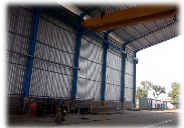
Overhead Crane (10 MT)
